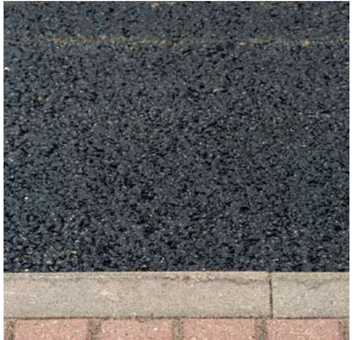
Asphalt Overlay
